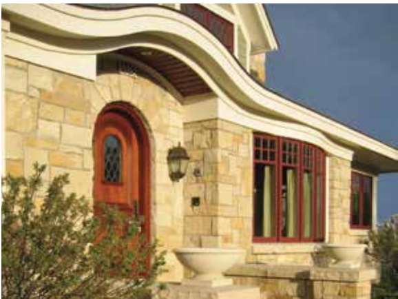
The barrel roof features Beaded InGrain Soffit
